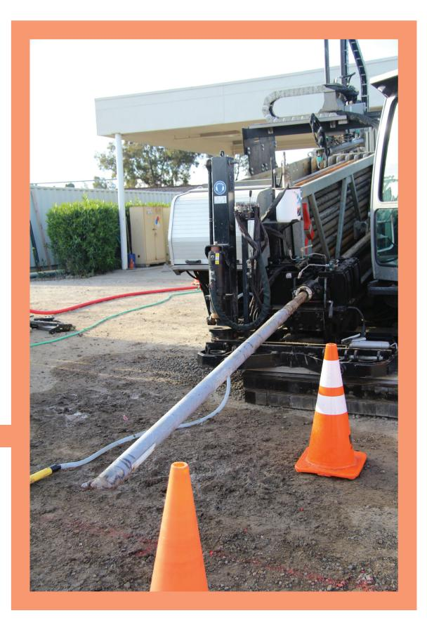
Coaxial cables, in the drill string enables high-speed communication, and power transfer, between the radar and surface equipment, over long distances
