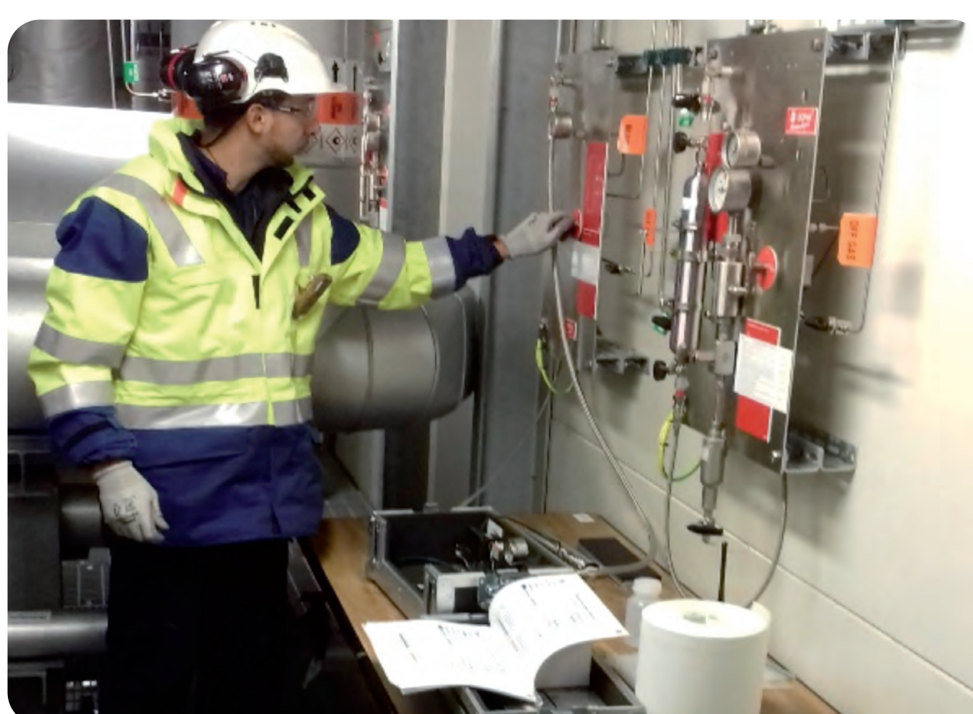
Operation at Gobigas
