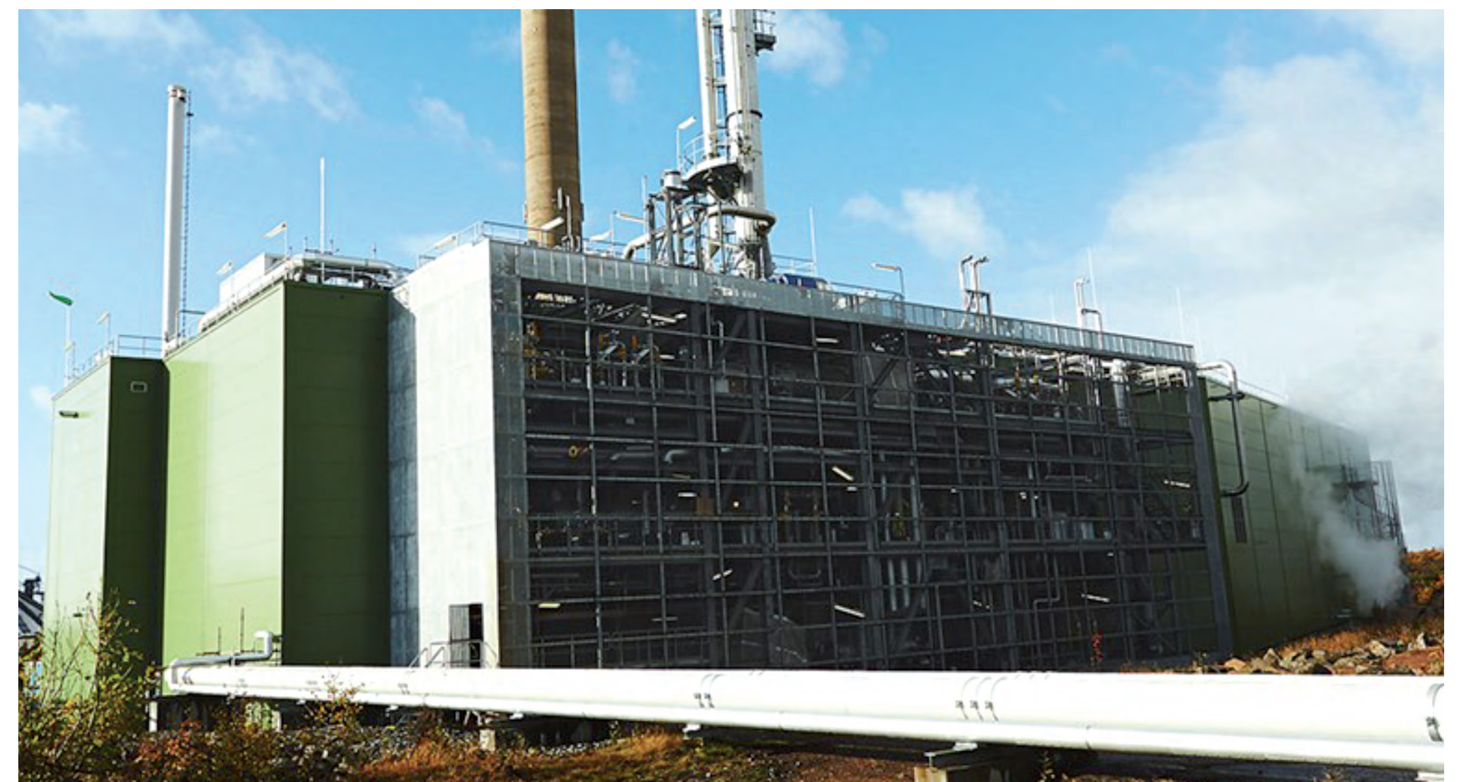
The GoBiGas facility
